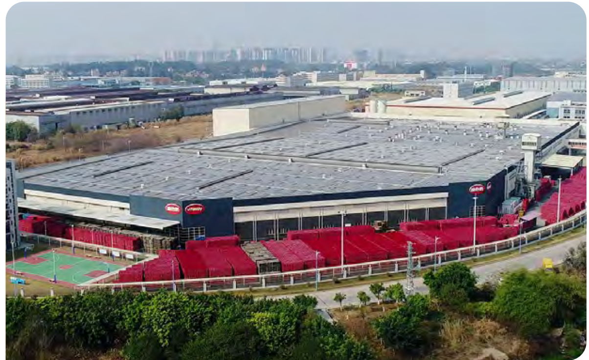
Rooftop solar panels at our Foshan manufacturing
